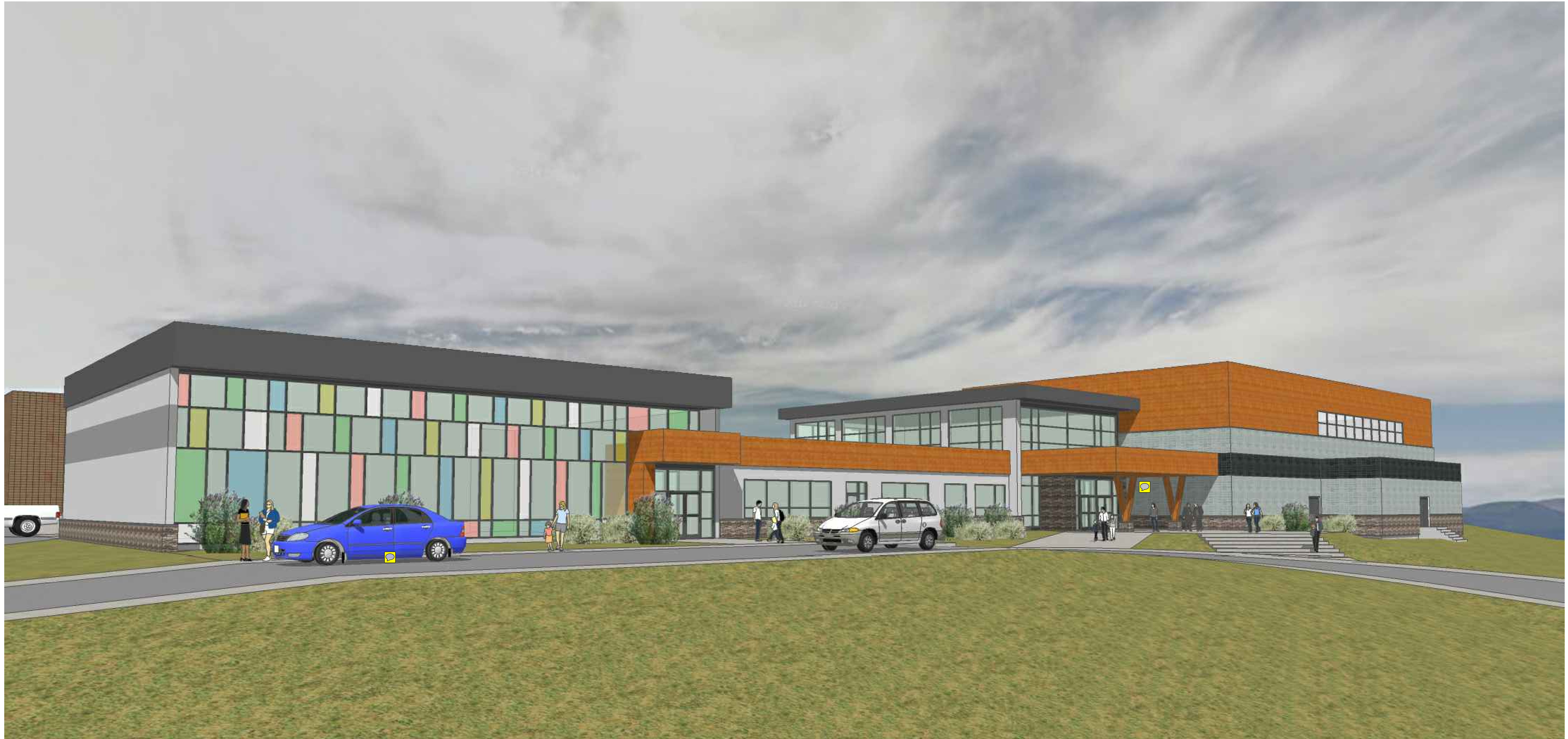
OVERALL VIEW TOWARDS SOUTH
